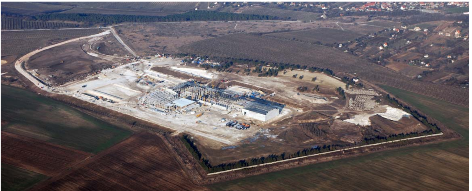
Aerial Construction Photo - Studio Complex
