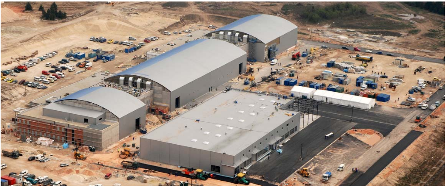
Aerial Construction Photo - Soundstages and Mill/Shops
