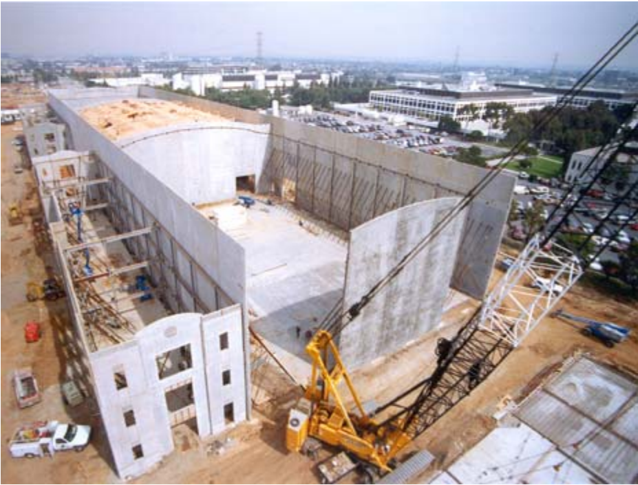
Aerial Construction Photo - Soundstages and Production Support
