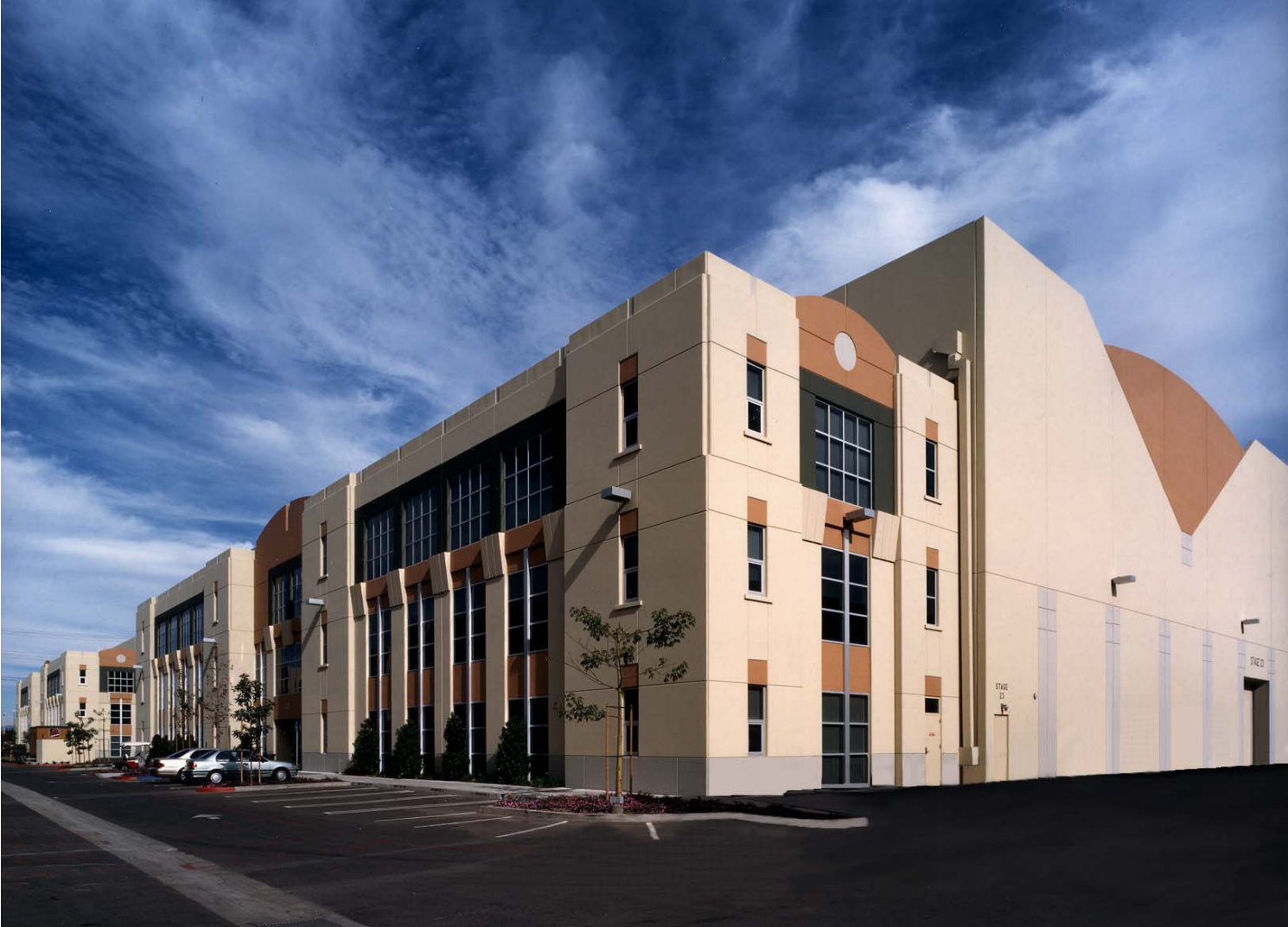
Production Support Building and Soundstage Beyond
